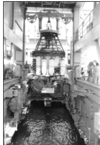
Figure 1-20. PTC Handling System, Elk River .
